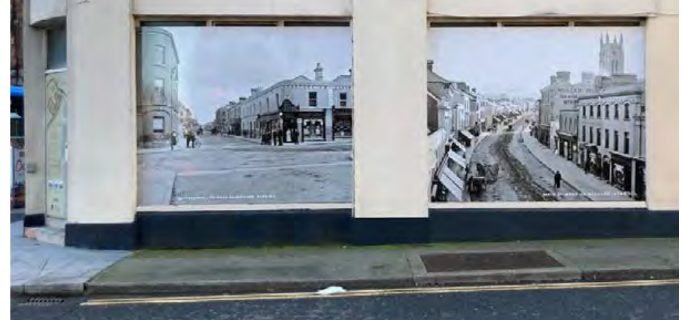
Right hand side windows, 110 Main Street - 2021
