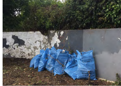
Heavy work at Alcove - 2020
