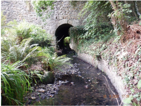
Plate 4-25: Swan River as it flows under Killarney Road (Site 6).
