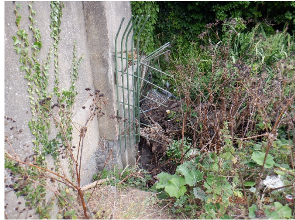
Plate 4-16: Pipe culvert where Swan River flows into Germans Wood
