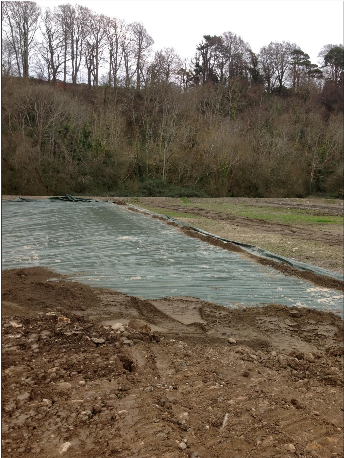
Plate 18. During the Dargle Flood Relief Scheme a large bund was constructed at The Slang to contain soil contaminated with invasive species excavated from the river banks.
