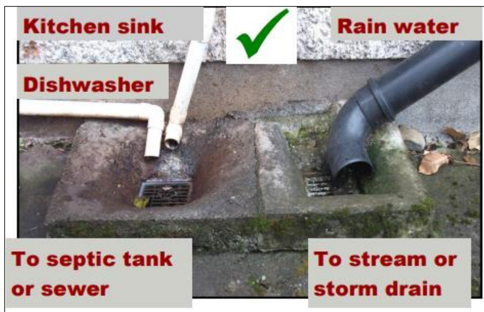
Figure 94. Correctly plumbed premises.
